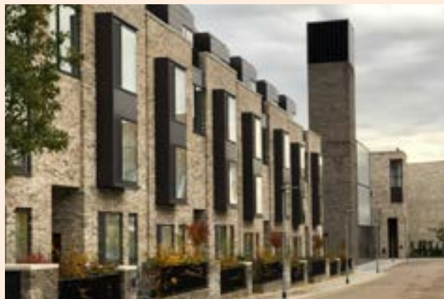
FIGURE 7: ENERGY CENTRE AT EDDINGTON, CAMBRIDGE, WHICH REUSES WASTE HEAT FROM SUPERMARKET FRIDGES TO SUPPLY THE LOCAL AREA WITH HEAT, AND IS INTEGRATED BEHIND SURROUNDING HOMES
